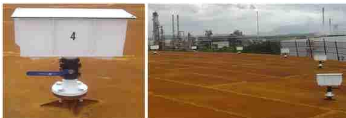
FIGURE 6. Dispensers installed on the tank tops
