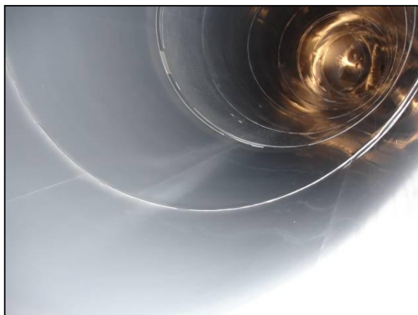
Figure 8- Inside view of the ECTFE liner
