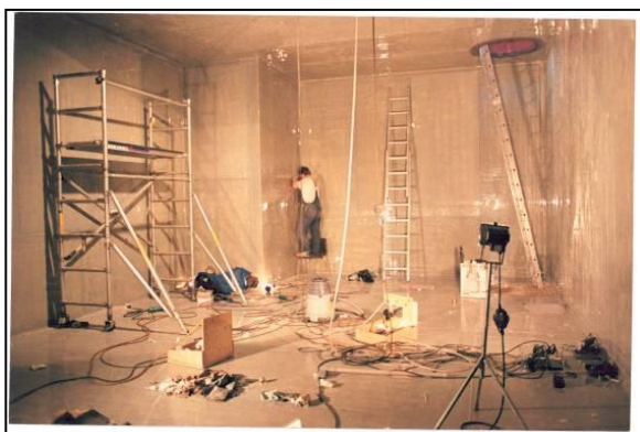
Figure 12 - Sheet lining of the tank, to be installed on the ship
