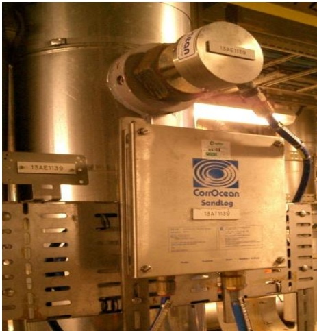
Figure 4: Sand probe and sand monitoring instrument for monitoring of vertical pipe.
