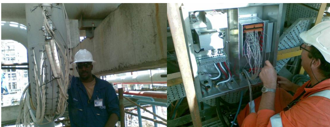
Figure 5: Installed sensing pins with field cables and termination in on-line instrument at the Jamnagar refinery site, India.
