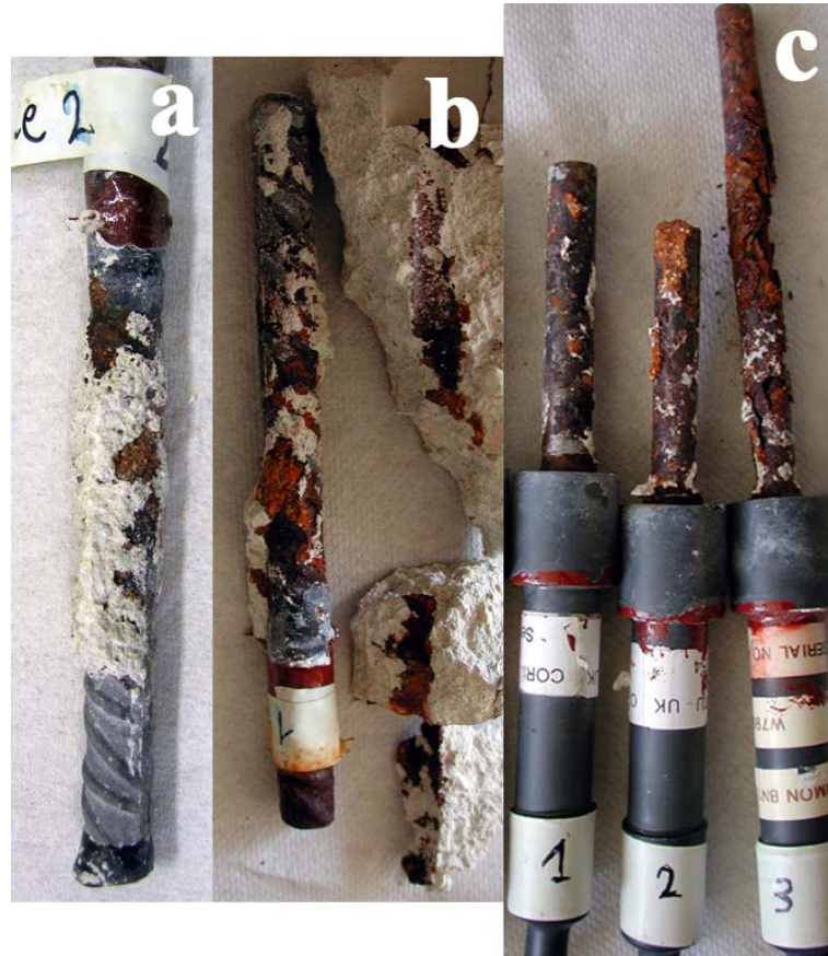
Fig. 10 - Corroded elements pulled out from CII specimen: rebars (a,b) and ERP probes (c).
