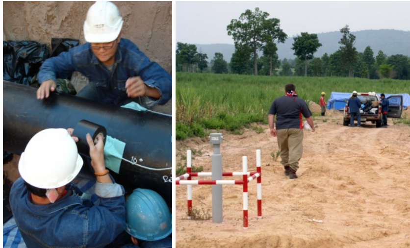
Figure 7 – Finishing the installation
