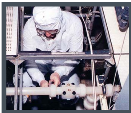
Photo 5 - Mechanically joined “Sanitary” PVDF piping system
