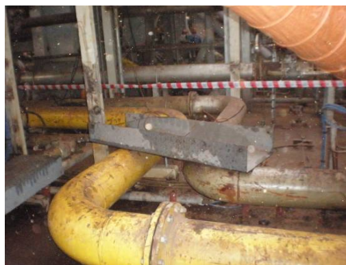
Figure.3: Example showing that blasting and painting of piping at workshop was of good quality. However paint work experienced a lot of mechanical damage, during transport and installation in addition to dirt on site.
